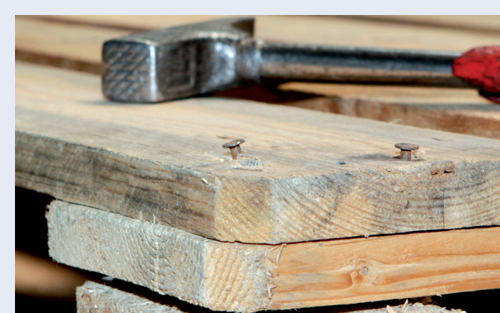
Hammering down projecting fastening elements
